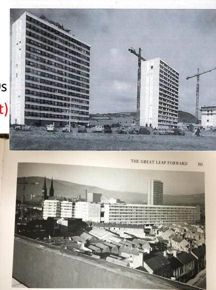
29.7. Belfast: NIHT's Area F1 Cullingtree Road Redevelopment Area ('Divis Flats'); 1970 view during construction by Laing, showing the 20-storey point block (Phase 1A) and several Sectra deck-access blocks (Phases 1B and 1B Extension) completed or part completed. (*Belfast Newsletter*)
